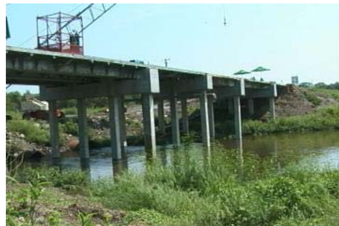
Railroad cars in place and welded together.
