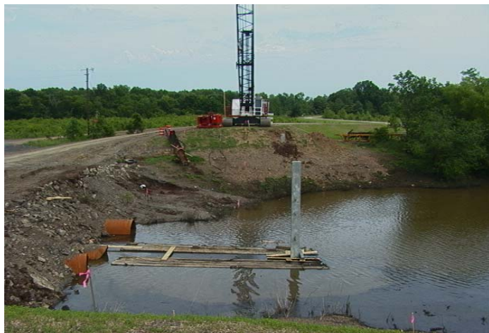
One piling driven, plenty more to go.
