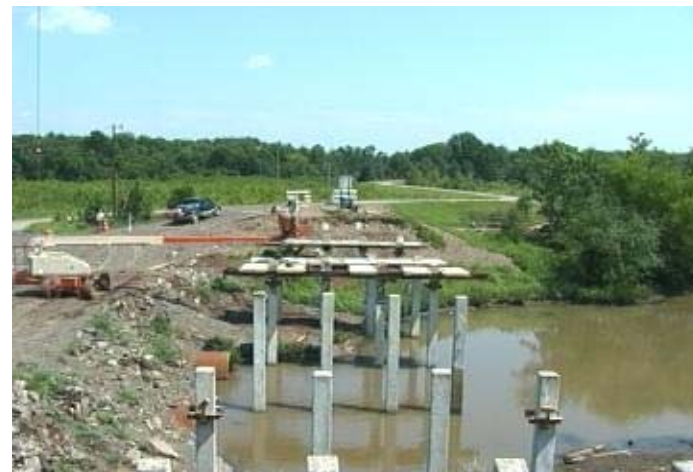
Pilings have all been driven, caps are being formed.
