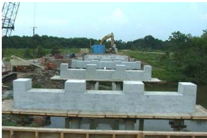
Caps have been poured and are curing before railroad car placement
