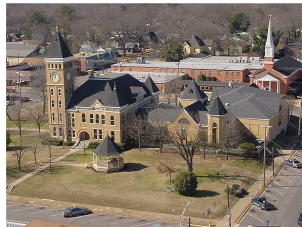
Saline County Courthouse, Benton, Arkansas
