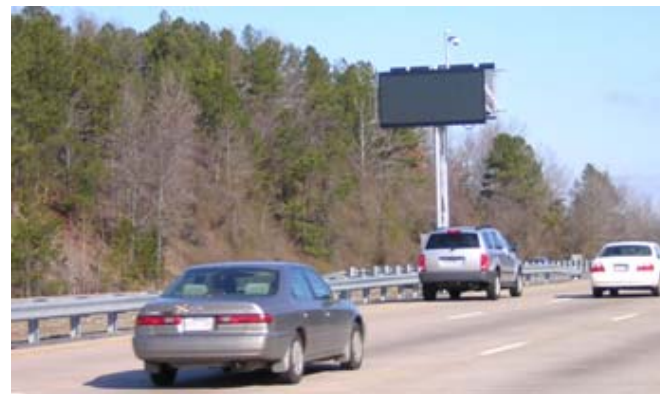
Interstate 430 in Little Rock
